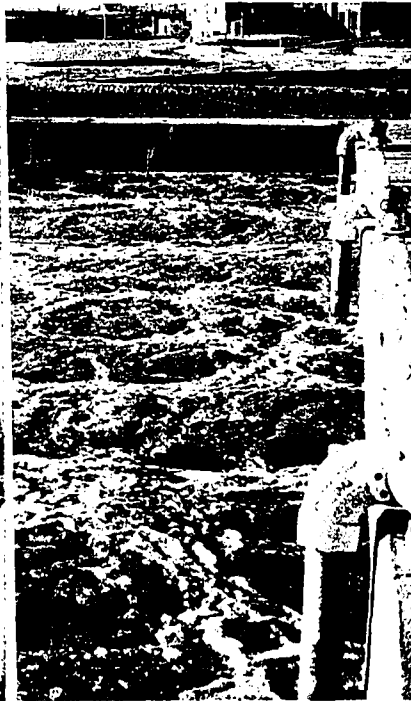
Fig. 59. Des Moines preaeration tank appearance at 2,000 cfm (0.10 cu ft/gal) aeration rate
